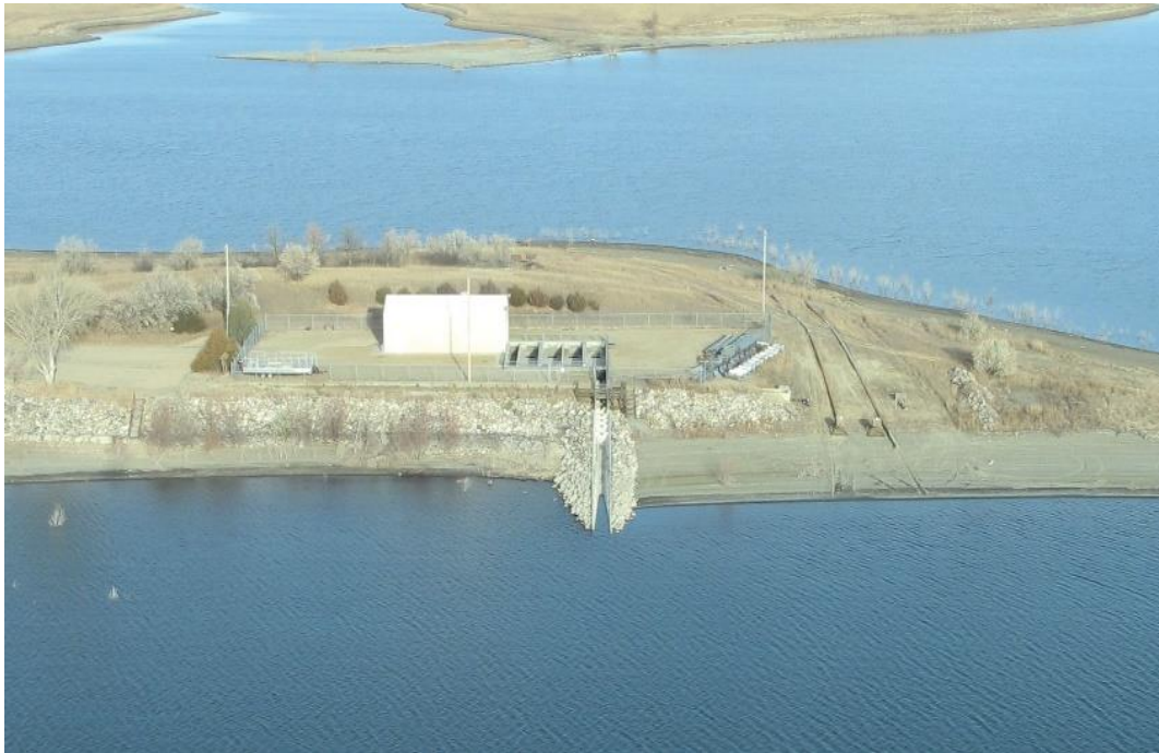
Figure 1. Aerial view of Whitlocks Spawning Station, Lake Oahe, South Dakota
