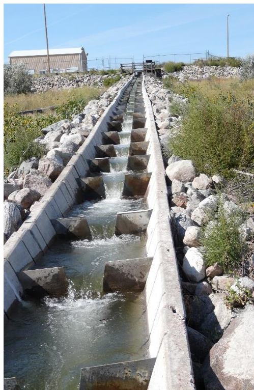
Figure 2. The fish ladder leading up into the catch raceway at Whitlocks Spawning Station, Lake Oahe, South Dakota
