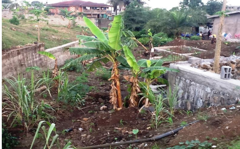
Figure 3. Valley Encroachment through Reclamation induces flooding of Chief Street Road Downstream during the Rainy Season
