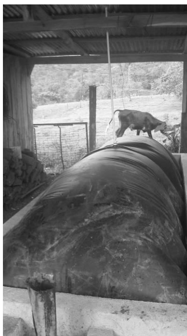
Figure 5. Biodigester System B – Media Salchicha
