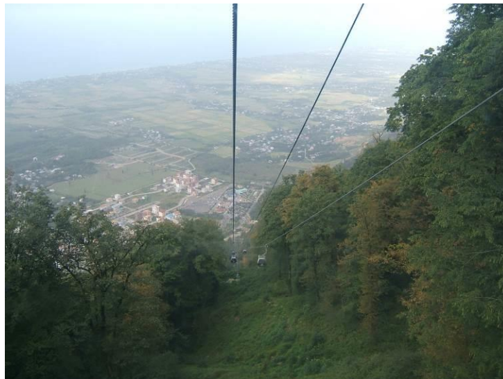
Figure 5. Namak Abrud has two cable car routes which transfer tourists from the main facilities in the village to the top of the mountain. It is evident in this photo that lots of trees have been cut in order to construct the cable car routes.
