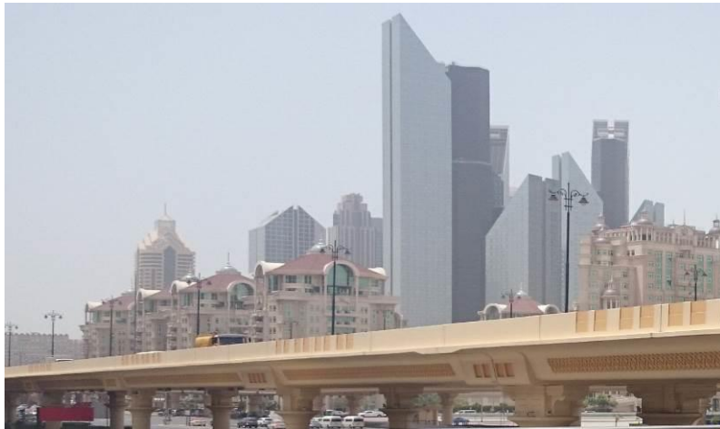
Figure 18. According to Emporis (2015), Dubai ranks fifth based on the number of tall buildings and skyscrapers after Hong-Kong, New York City, Tokyo and Chicago. There are currently 253 skyscrapers in Dubai (Emporis, 2015). The high rate of construction of new buildings in Dubai can cause environmental problems.
