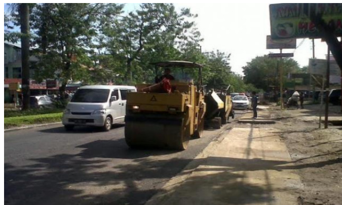
Figure 1. Before layer of road
