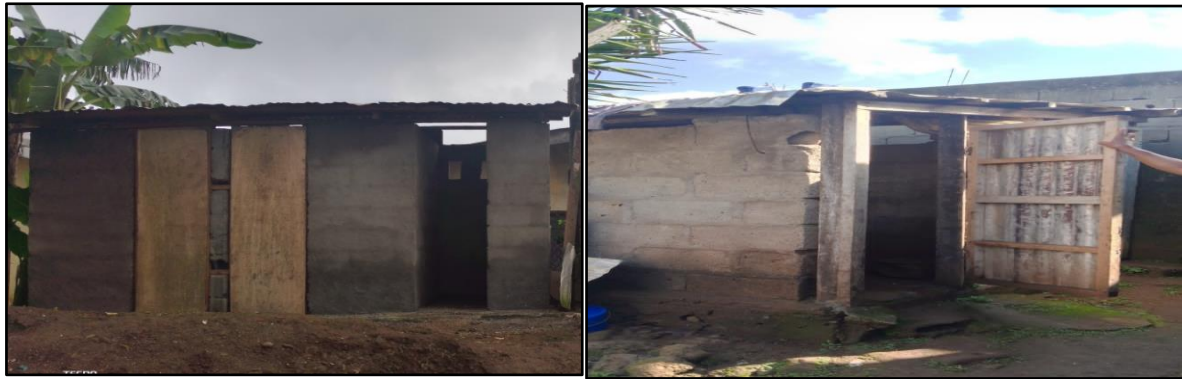
Latrines constructed out of cement bricks
