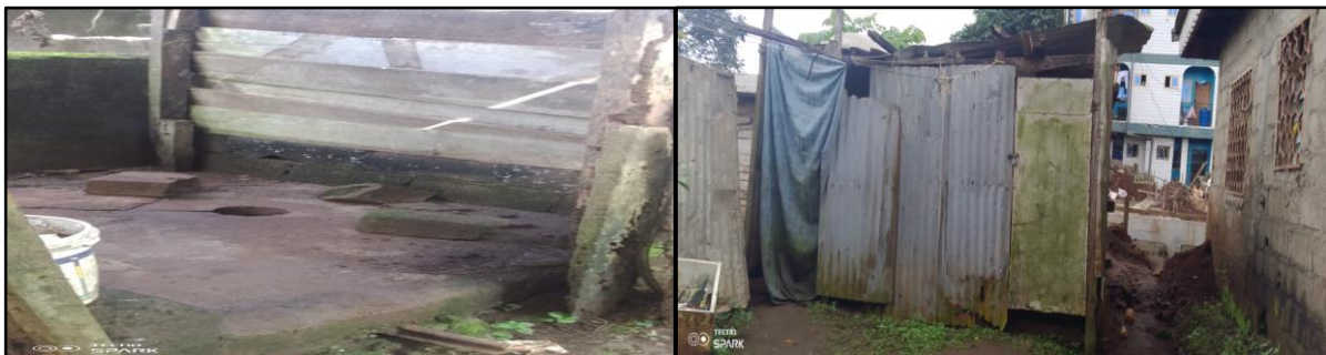
Latrines constructed out of plank materials
