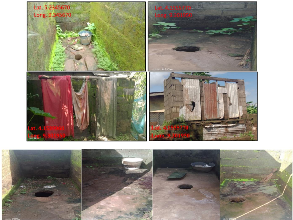
Plates 3: Evidence of dilapidated external and internal characteristics of latrines in Bomaka
