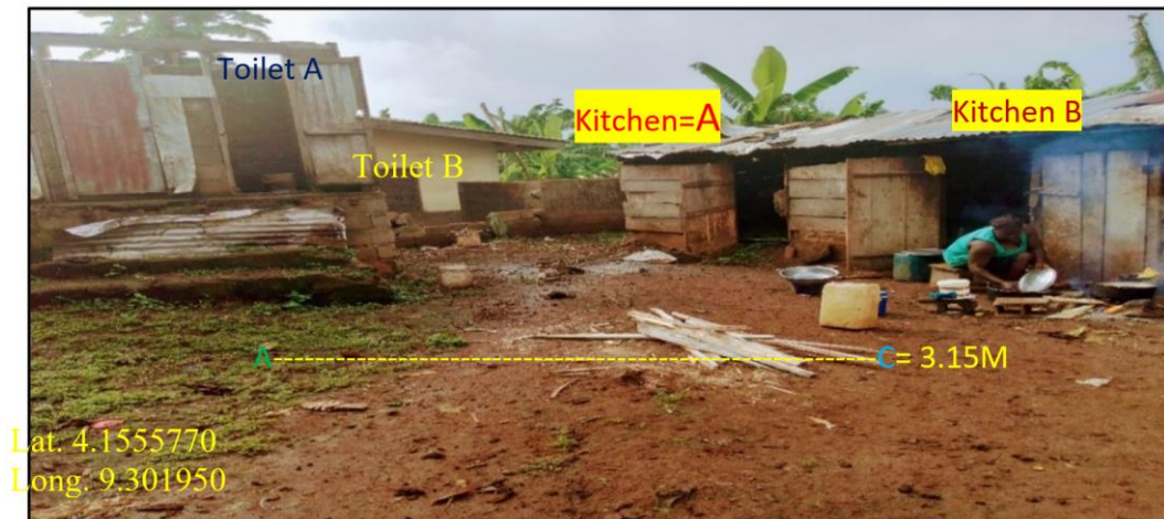
Plate 5: Vulnerability of some poor domestic kitchens located very close deteriorating latrines
