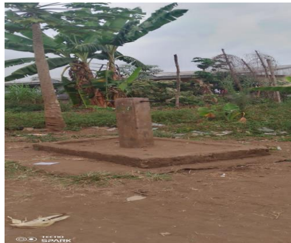
Plate 1: An abandoned water Tap in Bomaka
