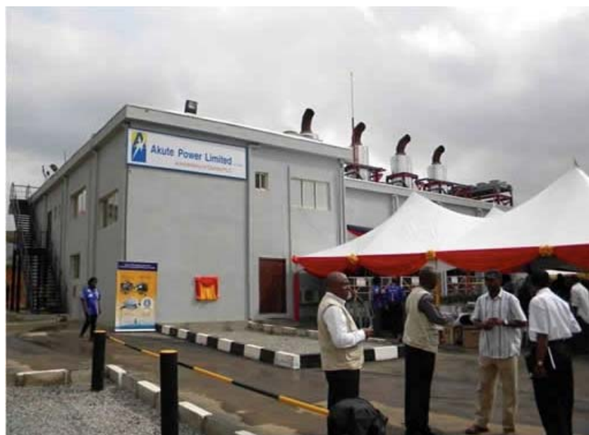
Exhibit 26. Akute Power Plant
