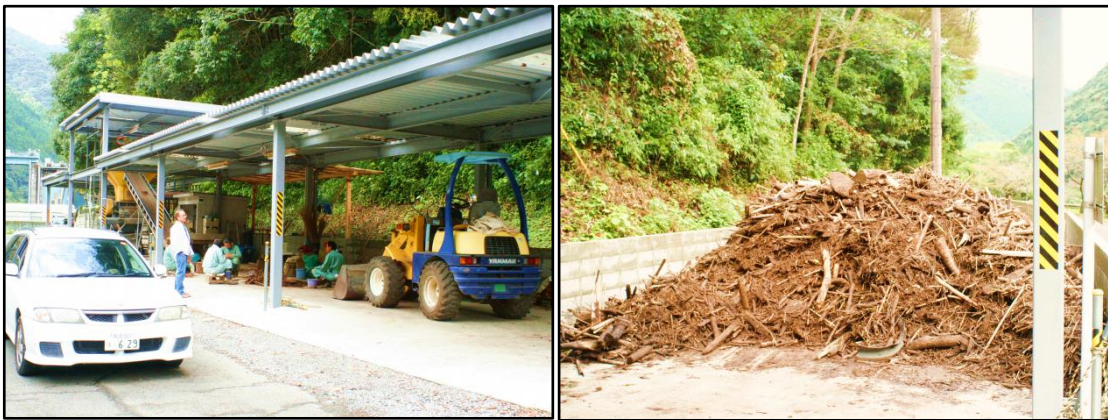
Figure 8. Removal of woody debris from the river above Setoishi dam. (Photograph by the authors)
