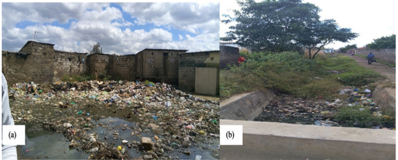
Figure 3. Showing a) Burning /indiscriminate waste disposal and b) Waste disposal in the drainage resulting in blockage of the drainage in Zone 98 of Kanyama Ward 10, Lusaka, 2018
