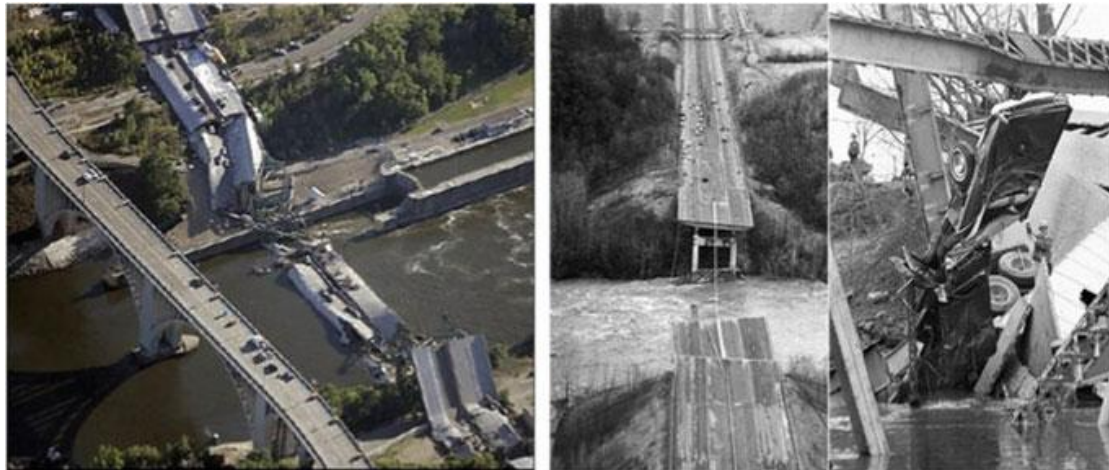
Figure 1: An example of Structural Monitoring Environment [17]
